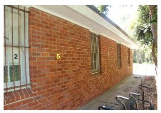
Figure 3.57 Western facade: Western facade of Buggy Store. Some of the windows were reused from the Stage 2 southern wing.
