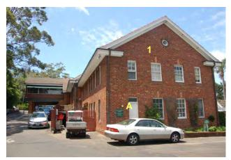
Figure 3.38 Northern facade: 'A' denotes a door converted from a Stage 1 window as part of the 1982 works.
